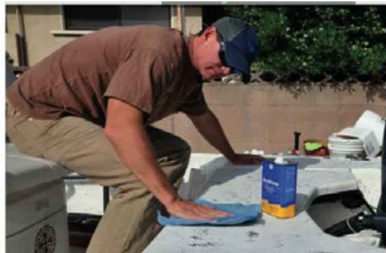
Clean surface with acetone and rag
